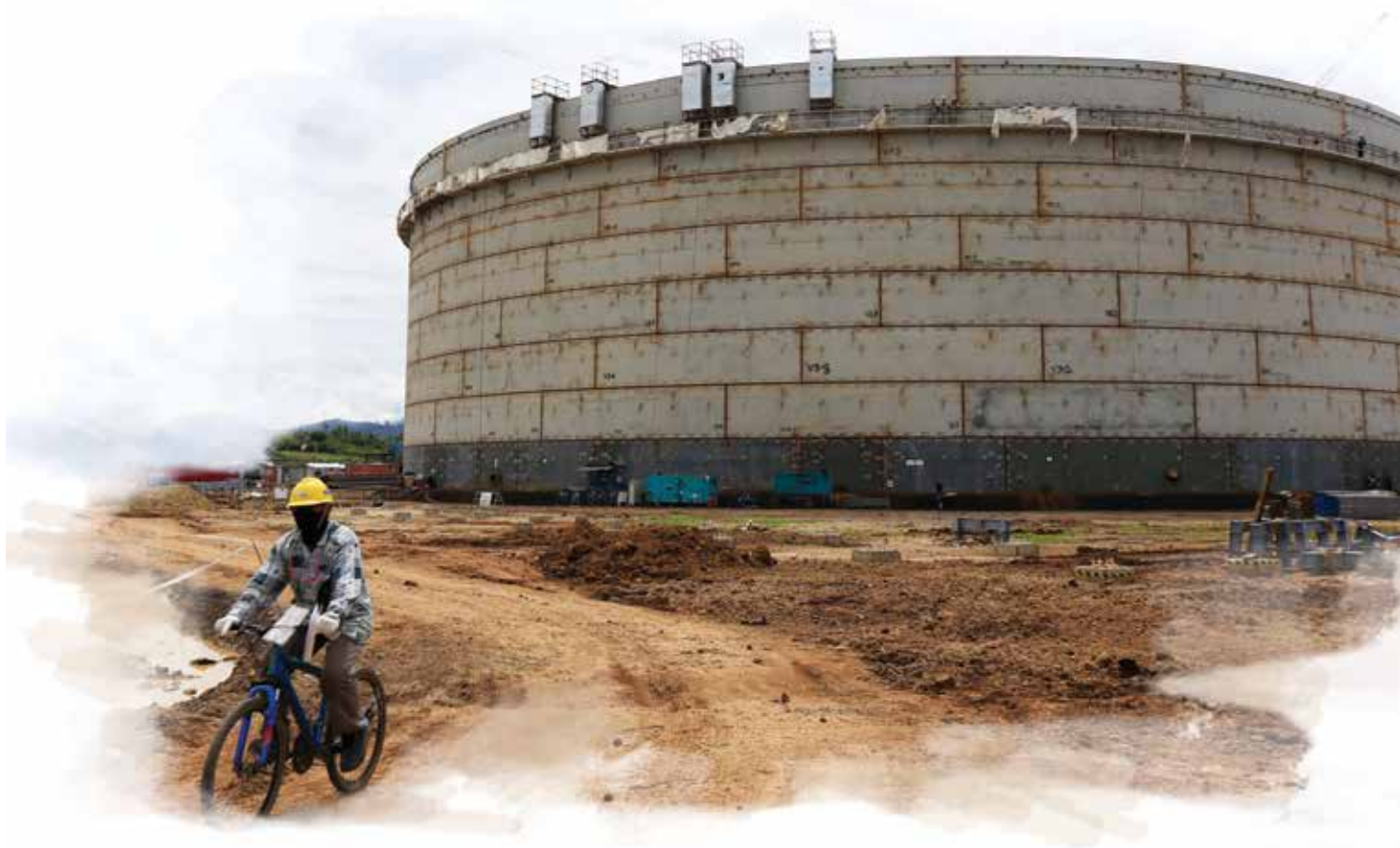
Konstruksi tangki Naphtha berkapasitas 60KT dalam proses Naphtha tank Construction of Naphtha tank with capacity of 60KT in progress
